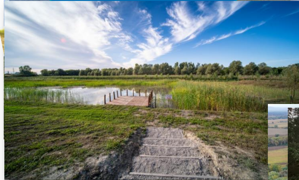
Multi-basin wetland to manage inland water inundation
